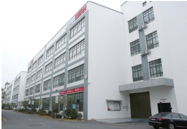
Portable Power Manufacture Base
